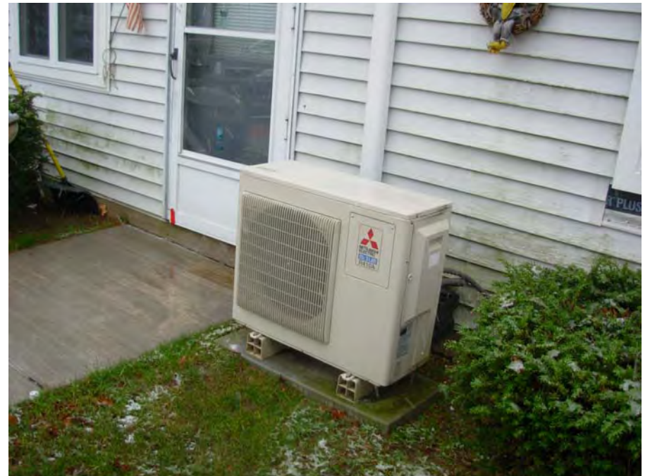
16. Heat pump condenser-compressor units at exterior
