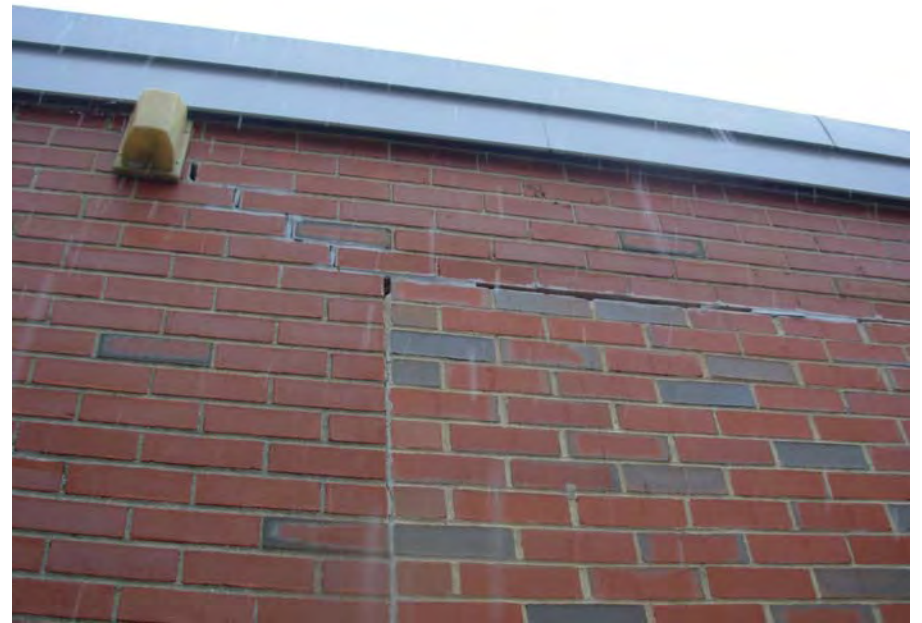
2. Minimal mortar deterioration observed
