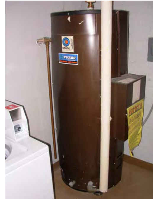
10. Original DHW serving laundry, to replace
