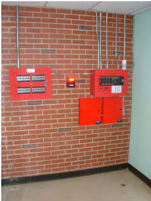
11. Fire detection-monitoring system, recently updated
