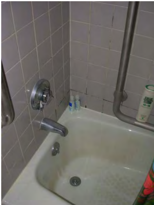
15. Tubs and surrounds, some to refinish - re-grout tile
